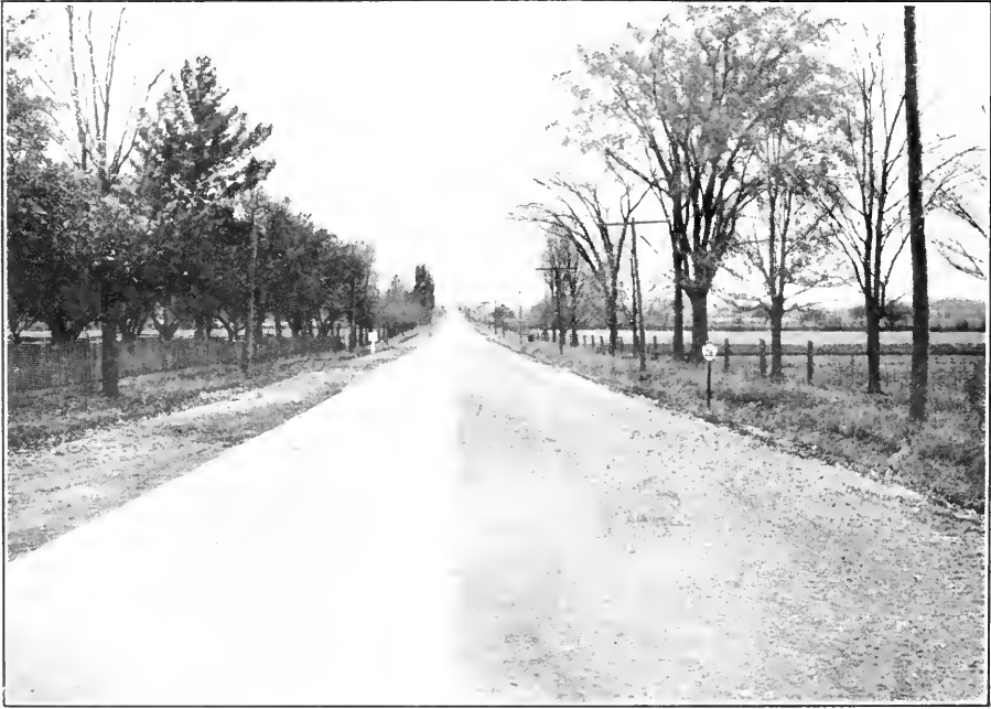
10' Concrete Pavement, Highway No. 26, East of Stayner.
